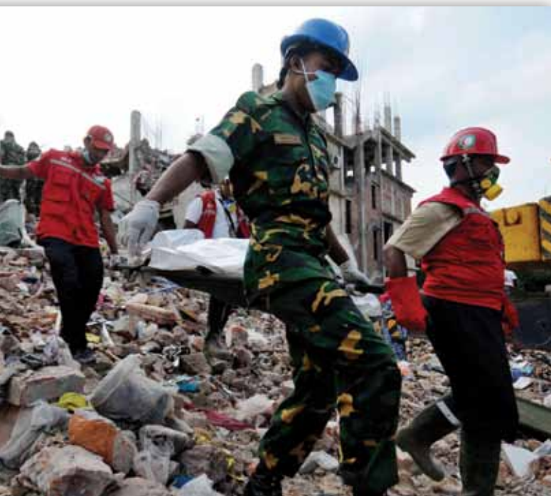
Rescue efforts for survivors in the Bangladesh continued a fortnight after the building collapsed
